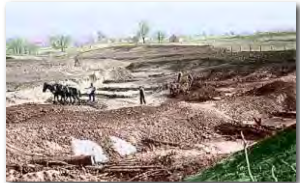
Brush dam construction on Chickasaw State Forest in the late 1930's to prevent further gully erosion
